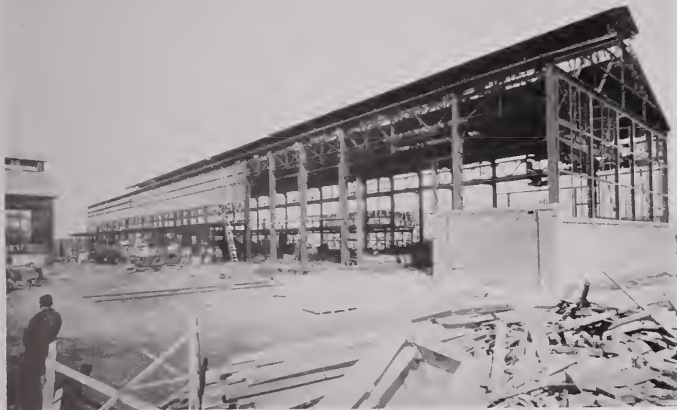
FROM THE SOUTHWEST
